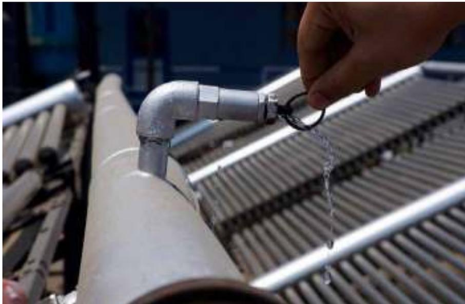
Figure 3 Vent valve to remove air from the collector circuit
