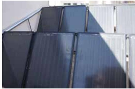
Figure 3 Collectors partly shadowed in the afternoon
